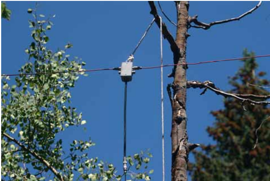
The NØLRA-designed dipole box in action.
