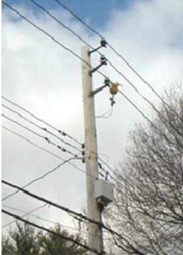
An Ambient BPL power-line connection in Briarcliff Manor. The yellow object is a tap off the medium-voltage primary. The gray cabinet holds the electronics. [Alan Crosswell, N2YGK, Photo]
