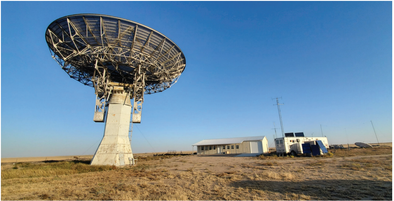
The larger 60-foot dish in the birdbath position. The pieces of the 30-foot dish are stored behind the trailer on the right.
