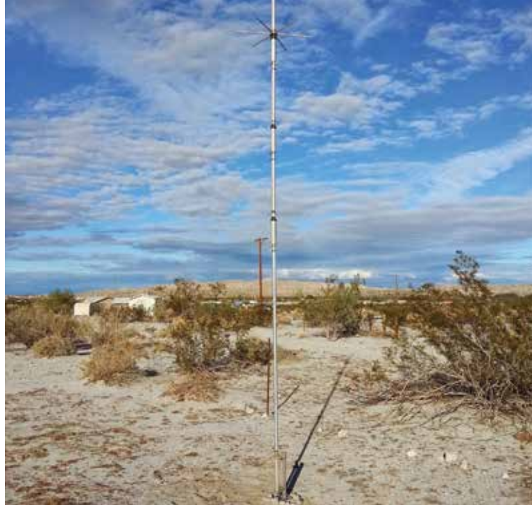
Figure 5: A multiband HF vertical antenna.
