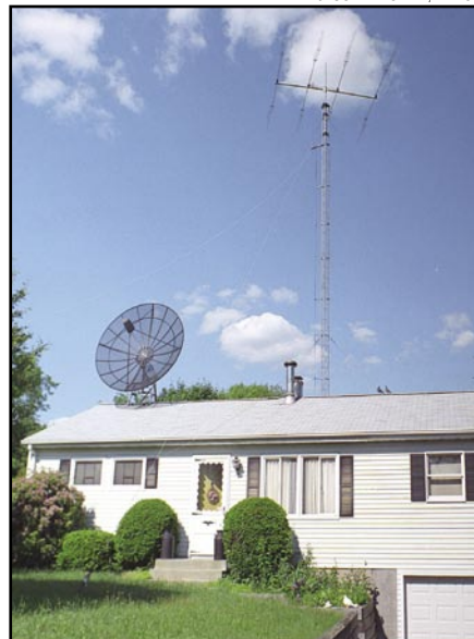
Brian Curtiss, AB1AI, of Wallingford, Connecticut, has a 65 foot Rohn 25 tower at his house. It supports a 4-element KLM KT 34A triband antenna for 10, 15 and 20 meters.
