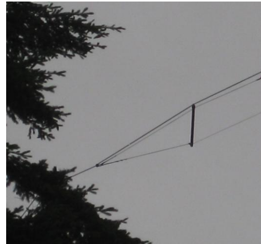
Figure 9. Detail of how both the parasitic wire and dipole are held taut by lines passed through remaining spacers to a loop in the catenary rope located about one spacer separation distance from the end of the dipole. As mentioned in the text, it would be better to keep the spacers away from the end insulators to avoid capacitive end loading, especially on the higher frequencies. This photograph is of a prototype 10 meter antenna. The photograph on the right is of W7ZZ's 40 meter dipole at 80 feet. For that prototype, a spacer was used as the end insulator for the dipole, which is why only one insulator is seen in the photo (for the parasitic wire).
